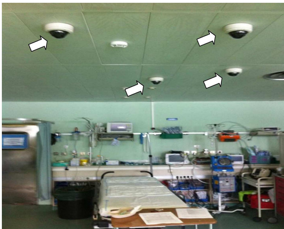
Figure 4 Distribution of video cameras in the Trauma and emergencies ICU of Doce de Octubre University Hospital (Madrid, Spain).
